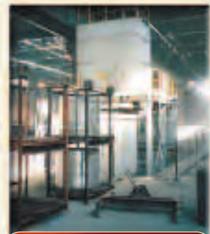
Aluminium Cable Solution Heat Treatment Furnace and Quench
