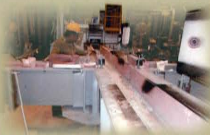
Interconnecting Launder System with Pre-heaters
